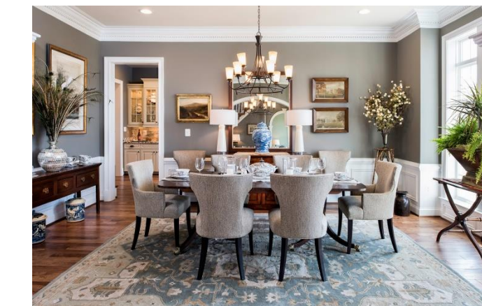
Dining room with box bay window, crown moulding, chair rail, and picture moulding
